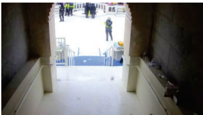
Image 2 (The “Tunnel” as seen on CCTV footage prior to rioters entering)
